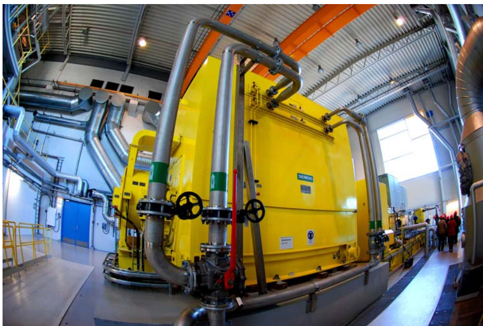
Picture: Electrical generator at Dåva 2 CHP, close to Umeå, Sweden.
