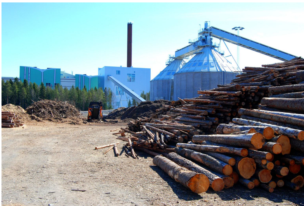
Picture: Dåva 2 CHP with storage silos and roundwood, Umeå, Sweden.
