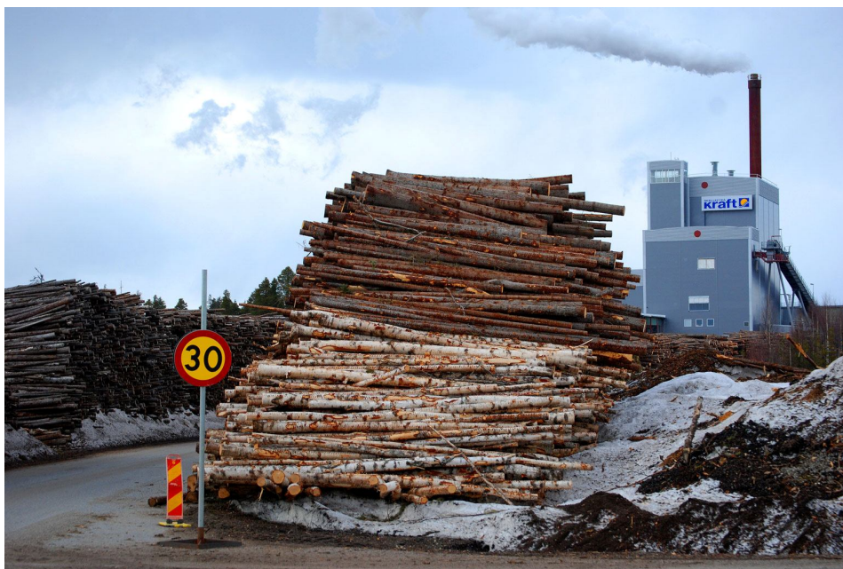
Picture: Skellefteå Kraft CHP in Lycksele, Sweden, uses roundwood.
